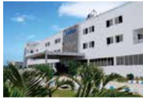
Rudrapur Plant (Green Building)
